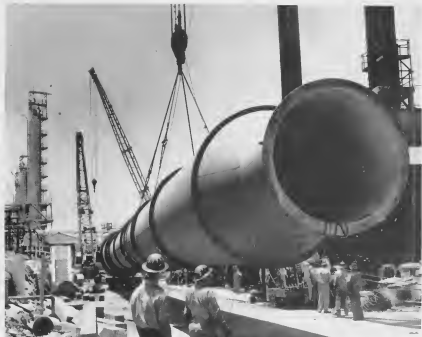
JUST BEFORE BIG LIFT, stack lies on side, lashings tight, load balanced, ready to be raised into place. POCO PROMER cu e trabao arandá a cuminsa, e staca ta na suelo, bon mara, balanza, eia pa worde hiza.
